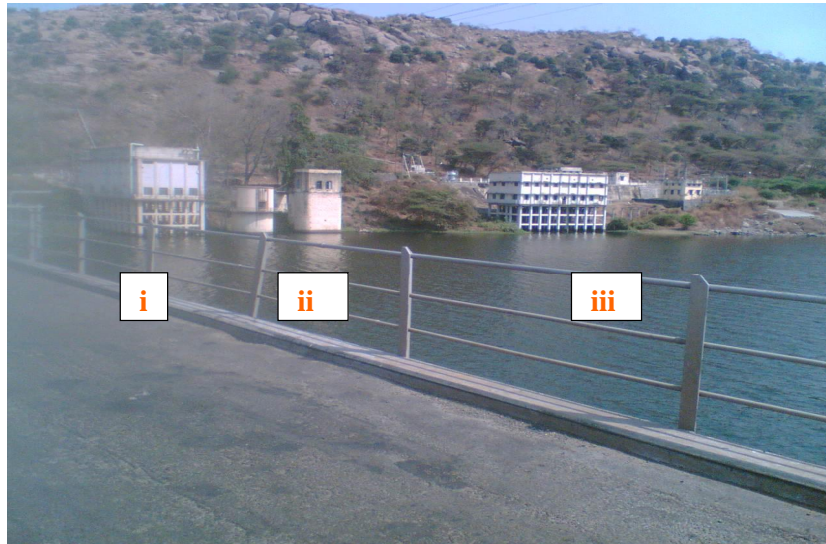
EXISTING INTAKE STRUCTURES IN THE RIVER CAUVERY NEAR METTUR DAM
