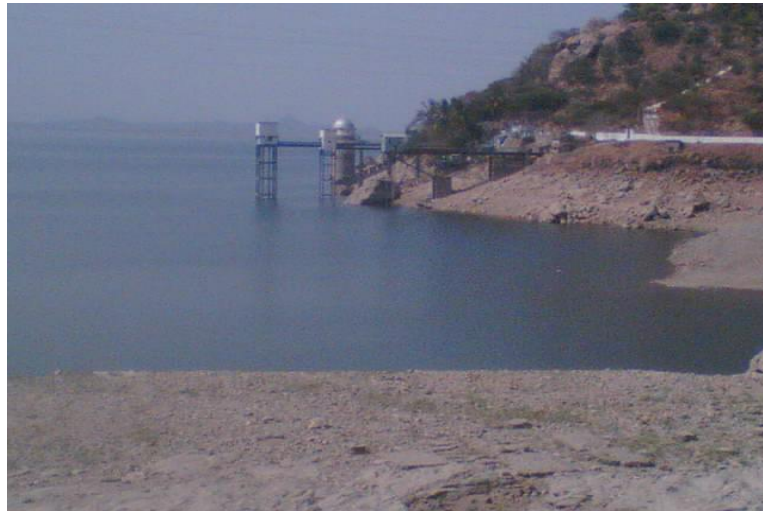
RAMAN INTAKE TOWER – METTUR SALEM SCHEME
