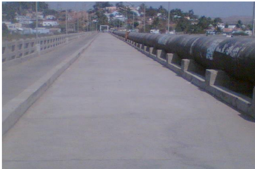
EXISTING PIPE CARRYING BRIDGE – SALEM ATTUR PROJECT
